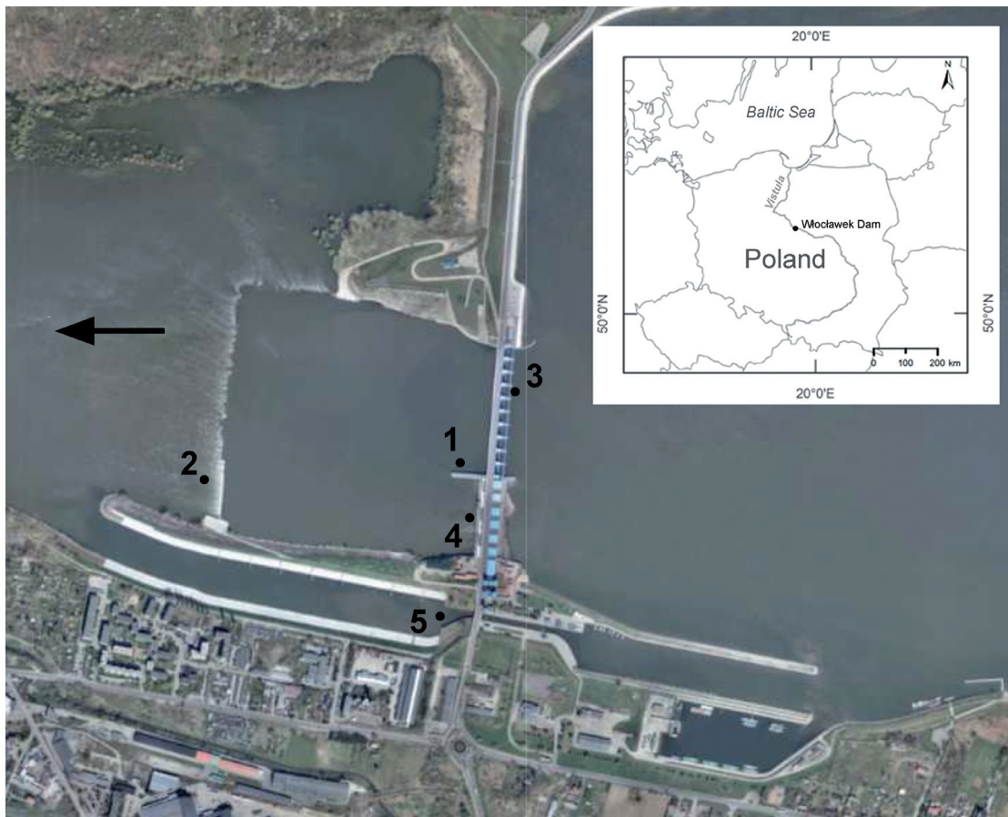
Figure 1. The location of the Włocławek Dam on the Vistula River. 1 = fishway, 2 = anti-erosion threshold, 3 = weir, 4 = turbine outlet, 5 = sluice, arrow = flow direction (orthophotomap under license from Head Office of Geodesy and Cartography, Poland).
